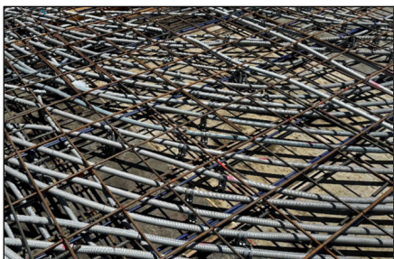
Fig. 3: A close-up of the reinforcement. Here, the top curtain of added reinforcement is more visible. Note from the shadows on the conduit that many of these appear to be within 1 in. (25 mm) of the reinforcing bar curtain
